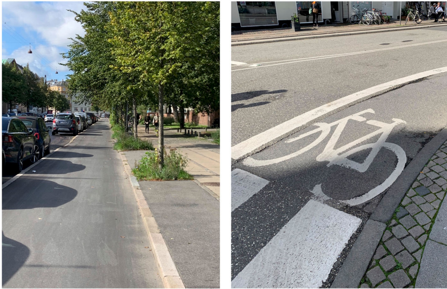
Figure 2. Types of bicycle infrastructure. The analysis includes dedicated bicycle infrastructure, which can be either protected bicycle tracks (left) or unprotected bicycle lanes (right).
